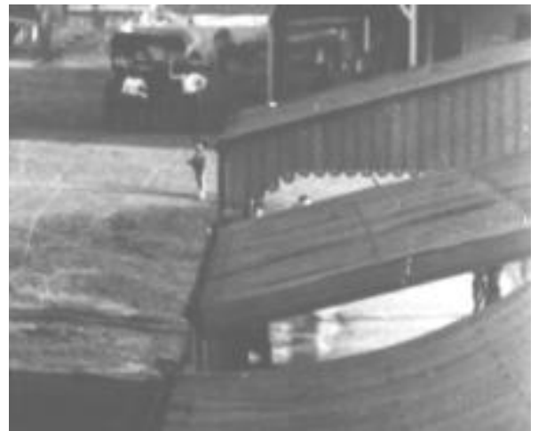
Figure 9. Examples of tongue and groove spandrel ends on awnings and parapet wall capping, lean-to and concave awnings.
